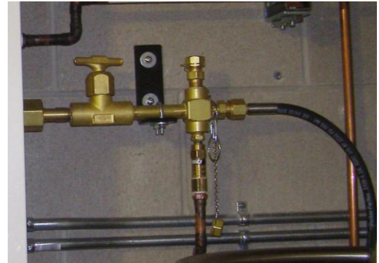
20" header length (Header pictured above accommodates 2 - 72" flexible pigtails for 2 portable bulk vessels + relief valve with pipe away)
